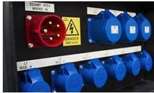
**Color Coding:** The Amphe-309 industrial connector's casing is color coded according to voltage and amperage ratings. In industrial situations where there are a lot of connectors mounted to a junction box (See image on left), the color coding of connectors is a decided advantage as far as operational readiness and maintenance convenience goes.
